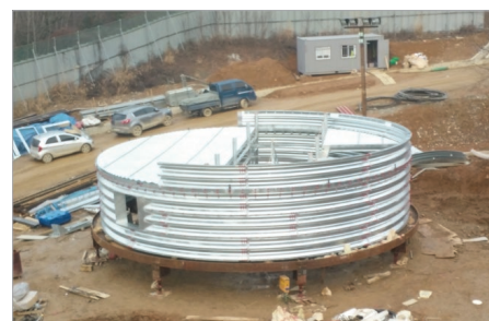
[3. Outdoor production of corrugated steel pipe]
