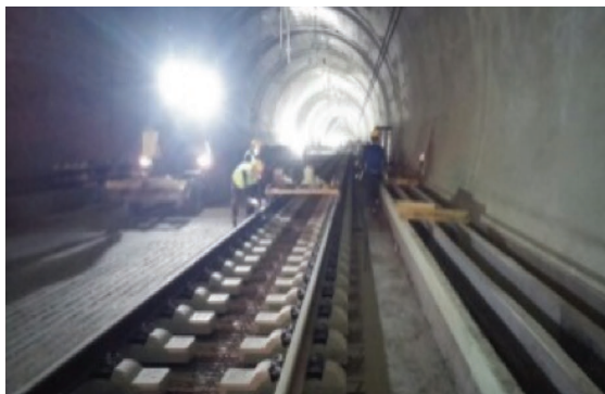
[Temporary installation of rails]
