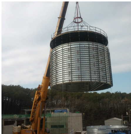
[4. Lifting corrugated steel pipe]
