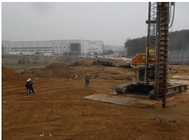
[1. Site clearance and H-pile driving]
