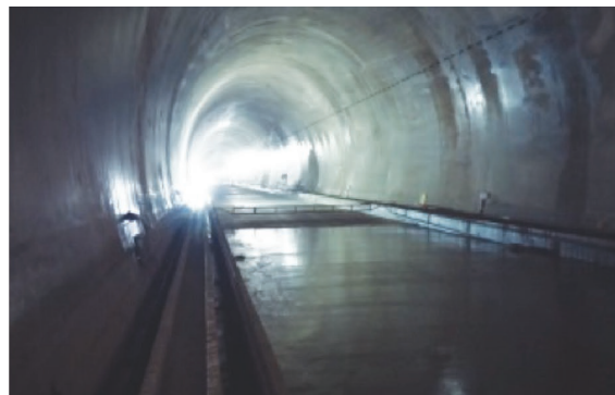
[Installation of structural elements for the main tunnel]
