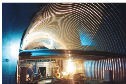
[2. Slab installation to create two floors within an adit]
