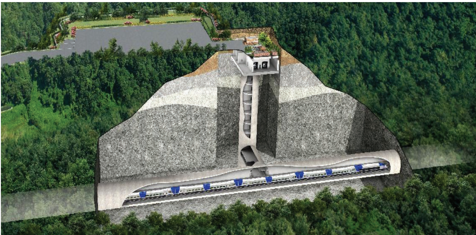
[Image of a 74-meter-deep vertical shaft adjacent to the main tunnel]
