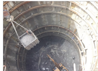
[3. Blasting and earth removal at vertical shaft]
