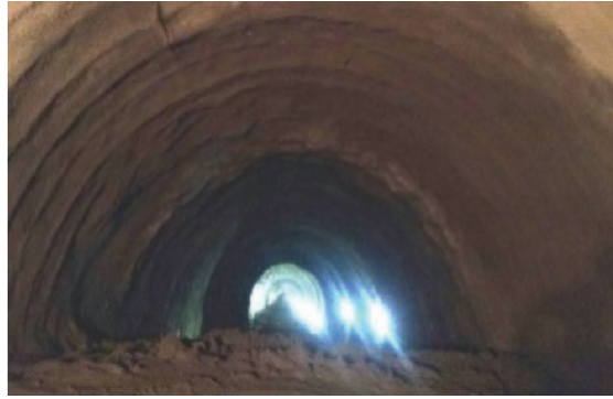
[Tunnel excavation and penetration]
